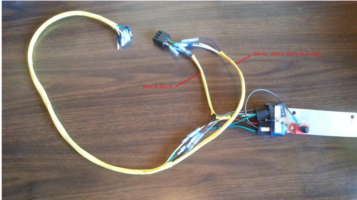
Figure 23 Bench test using new harness.
