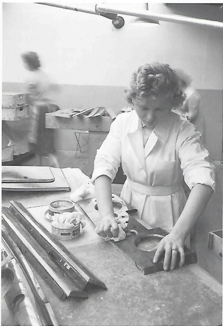
A typical wooden dashboard being French polished, prior to being fitted into a Mk I 2.4-litre saloon. (Courtesy Jaguar Daimler Heritage Trust)
